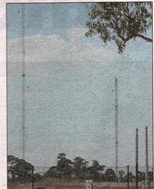
Masts from past: The former Radio Australia site at north Shepparton is the only radio transmission site in Australia where the original broadcast towers are still standing.
