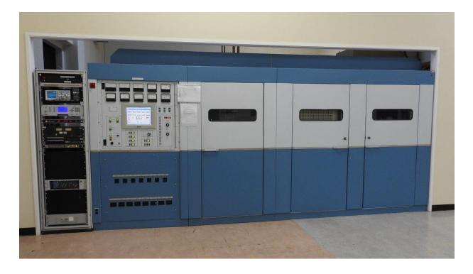
The Continental 418G 100KW AM/DRM transmitter at Radio Australia. This transmitter was installed around five years ago. DRM is Digital Radio Mondiale, a form of short wave digital radio transmission. It has not become popular and this transmitter has not been used in this mode to my knowledge.
